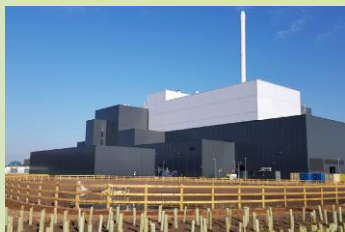
Waste to Energy
