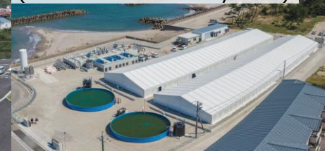
Onshore Aquaculture Plant (Water Treatment System)
